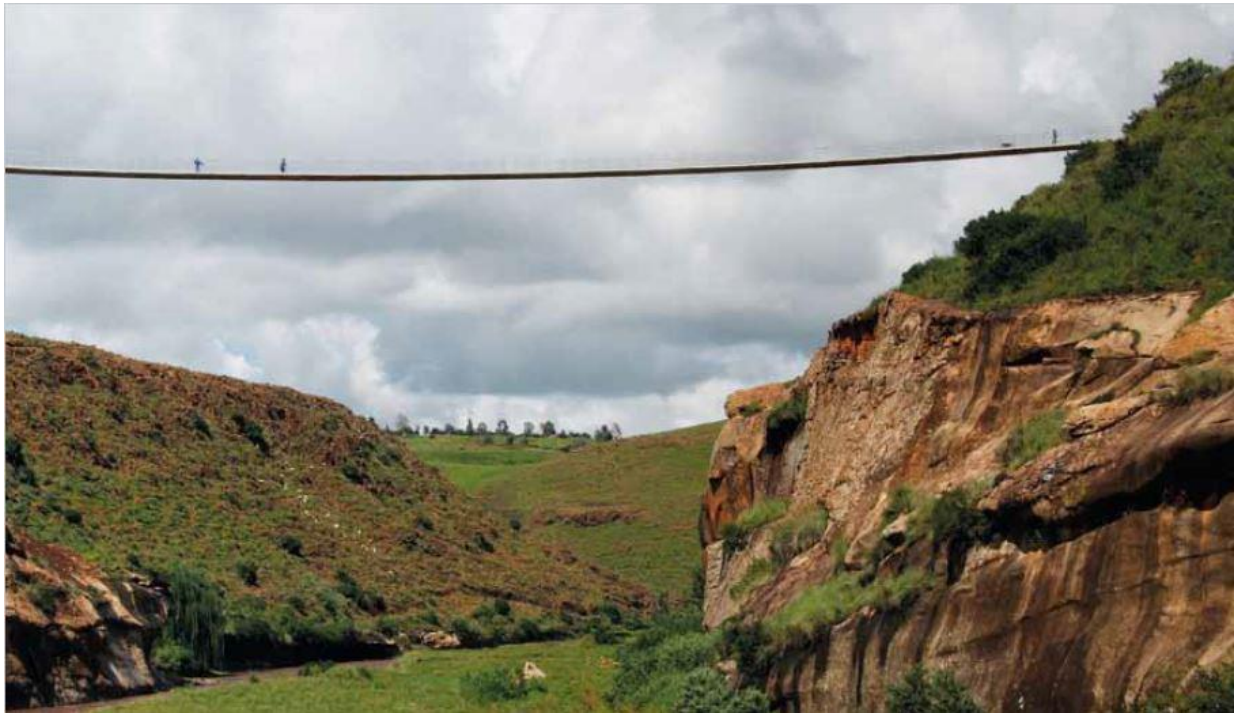
Figura 4.25 – EXEMPLO DE “STRESS RIBBON BRIDGE” 31
