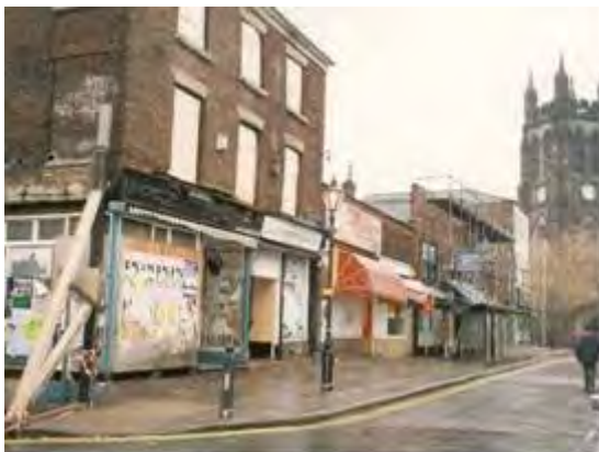
Staircase House before
