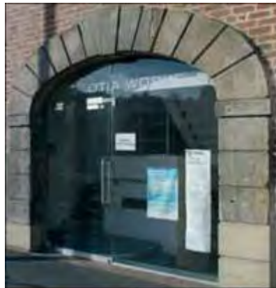
Scotia Works after
